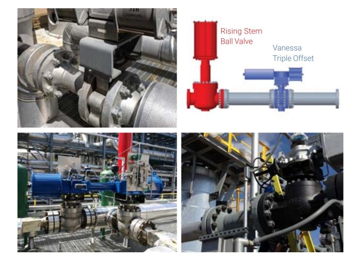
Emerson's AE valves provide a high-performance replacement for rising stem ball valves, offering a more compact, reliable, and cost-effective solution. With fewer moving parts and double-eccentric technology, AE valves reduce maintenance, improve sealing performance, and enhance actuation efficiency. Backed by Emerson's expertise, they optimize positive shutoff while minimizing downtime and operational costs.
